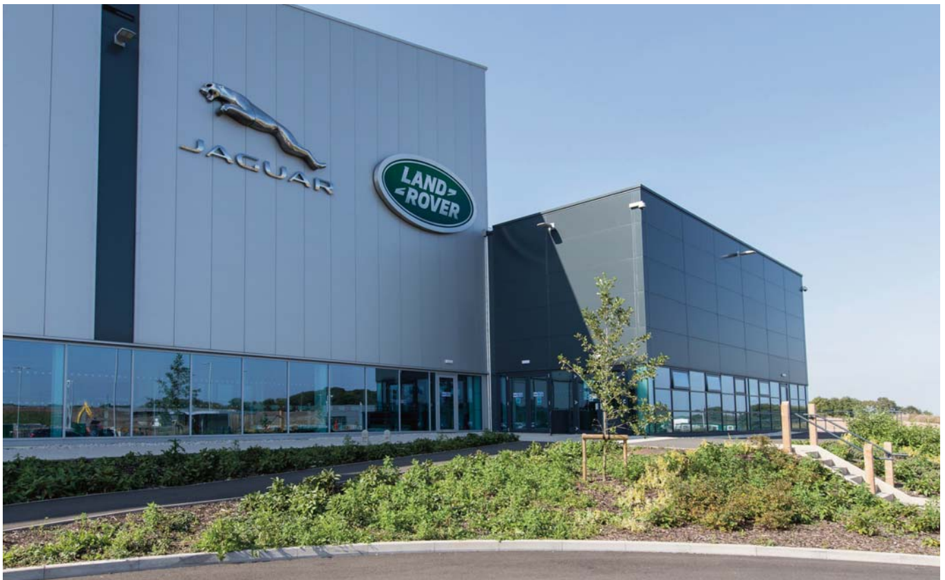
Jaguar Land Rover's new Engine Manufacturing Centre at the i54 Business Park
